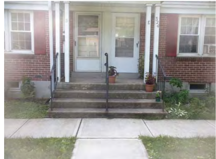
Concrete stoops at the front and rear door to each unit are in fair overall condition
